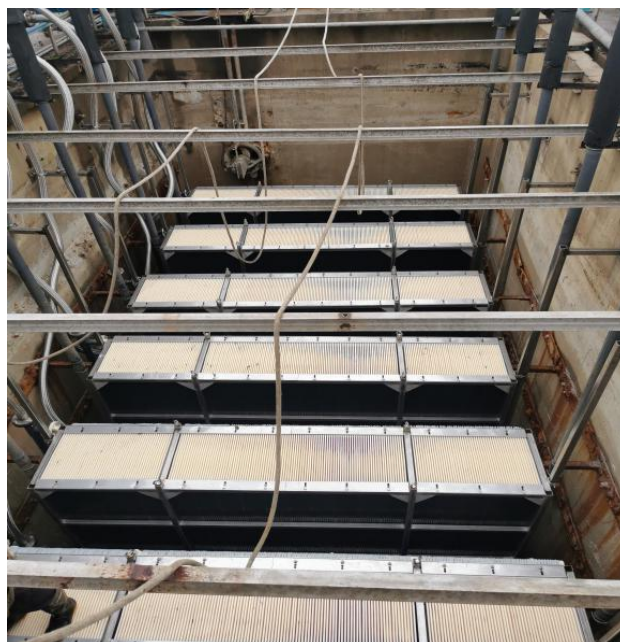
3S membrane module as a replacement
