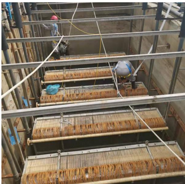
MBR flat membrane'd been running for 5 years
